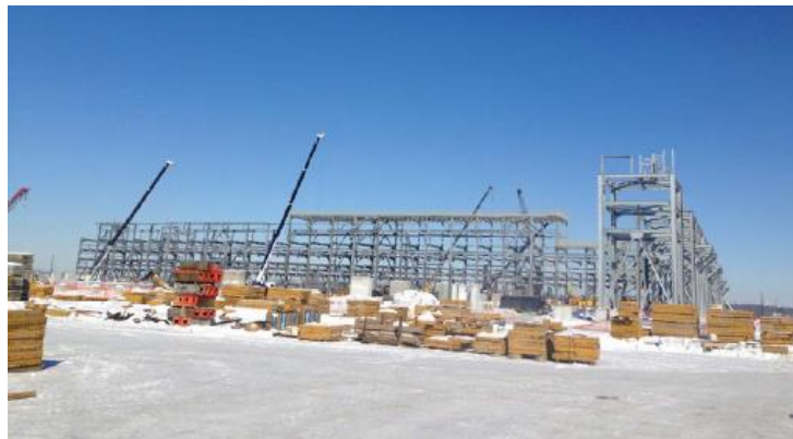
Ammonia steel structure erection
