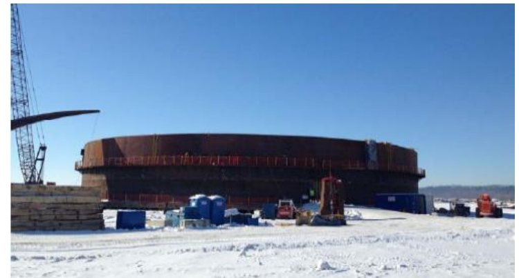
Ammonia tanks shell rings installation
