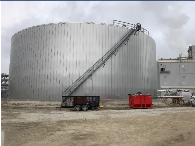
Newly Added Diesel Exhaust Fluid Tank in Iowa
