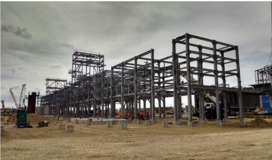
Pipe Rack Erection
