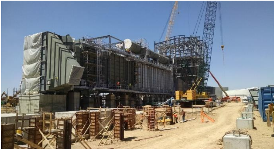
Reformer Box Erection
