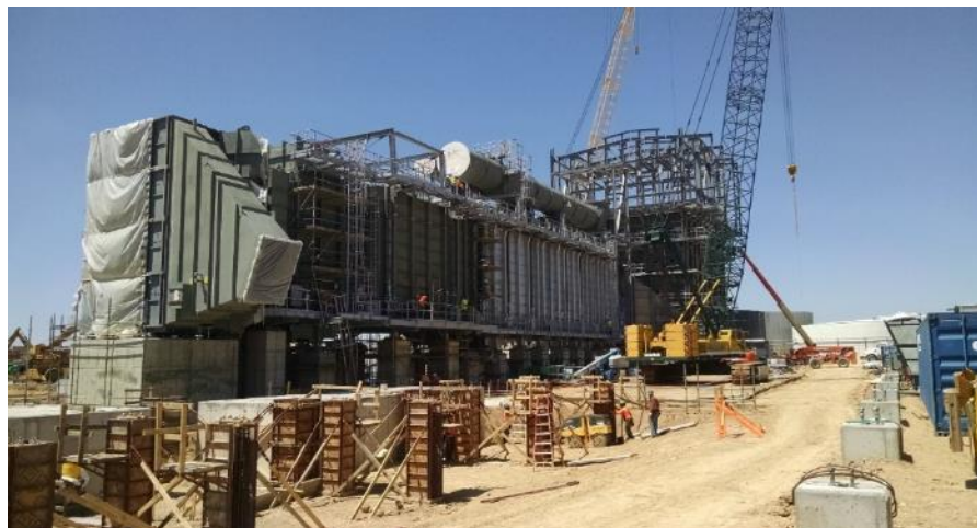
Reformer Box Erection
