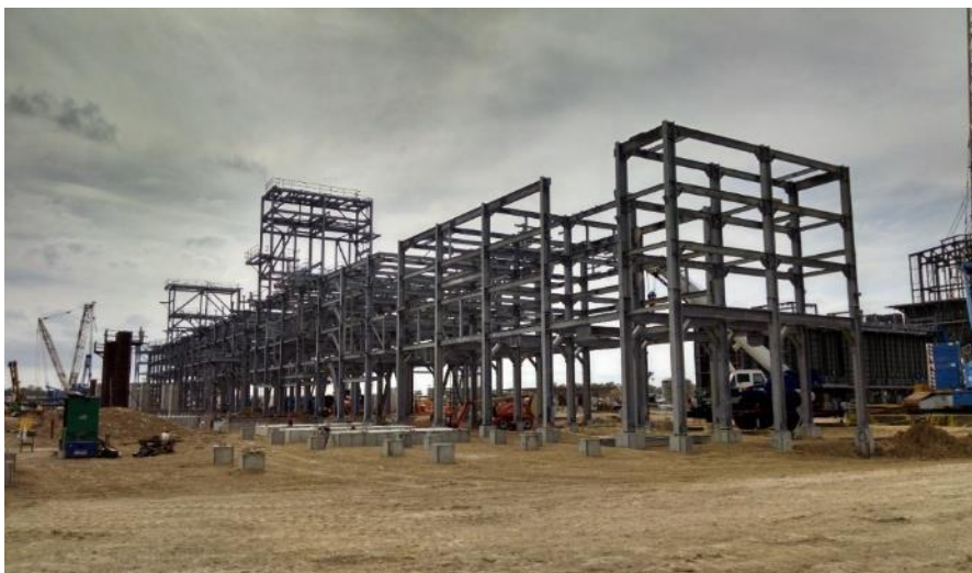
Pipe Rack Erection
