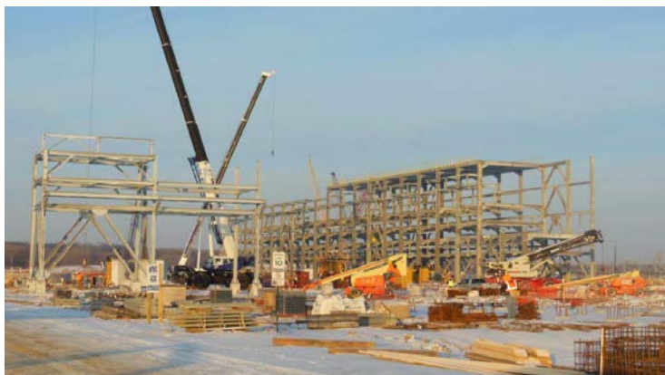
Ammonia pipe rack steel structure erection
