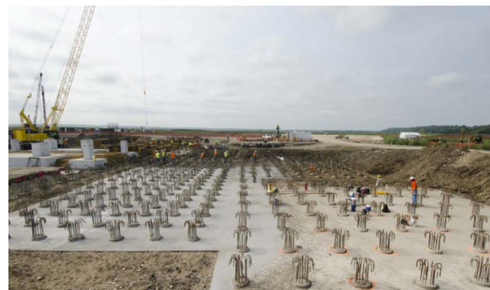
Reinforced concrete foundations
