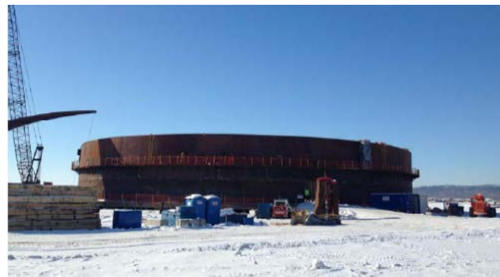
Ammonia tanks shell rings installation
