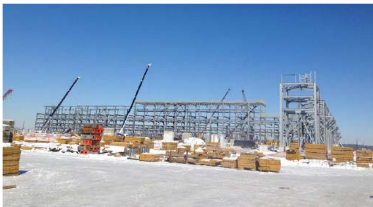
Ammonia steel structure erection
